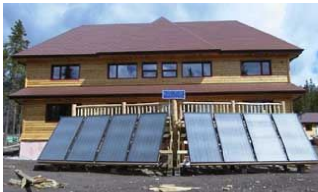
Architectural solar panel at the Aurum Lodge in Alberta, Canada. The panels provide shade during summer months and heat during the winter season.
